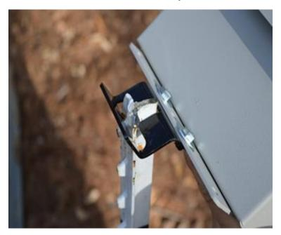
Align mount swivel ball stud using ¼-20 threads into the top solar mounting port. Thread ball stud no more than three complete rotations into solar mounting port. Tighten ball head adjusting nut securely to solar port. Do not over tighten.
