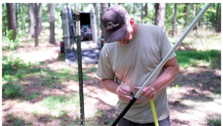
Loosely secure extended pole with nylon adapter to T-post with at least three zip ties. Ensure extended pole locking tabs are centered between T-post spine and stud base to allow later camera field of view adjustment.
